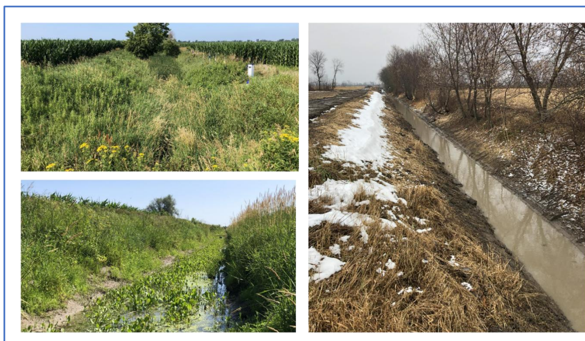
Figure 2: Agricultural drainage ditches, displaying wetland-type features. Clockwise from top left: ditch prior to dredging; ditch after brushing of woody vegetation and dredging; ditch regeneration post-brushing. (© Agriculture and Agri-Food Canada)
