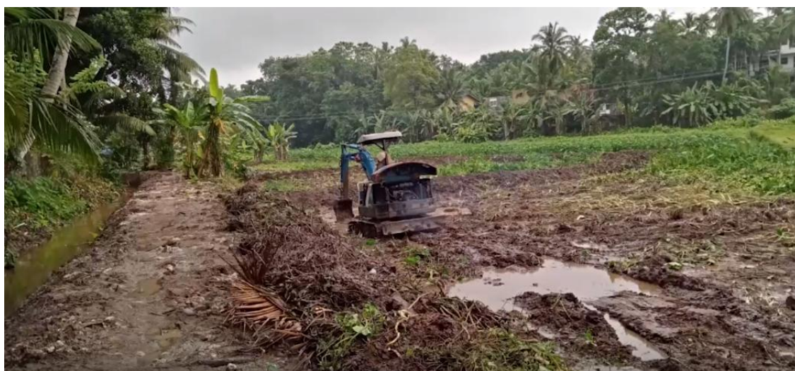
Figure 3. Cleaning and excavation of degraded paddy fields and canals. (© Padmini Perera/Manosha Welikala)
