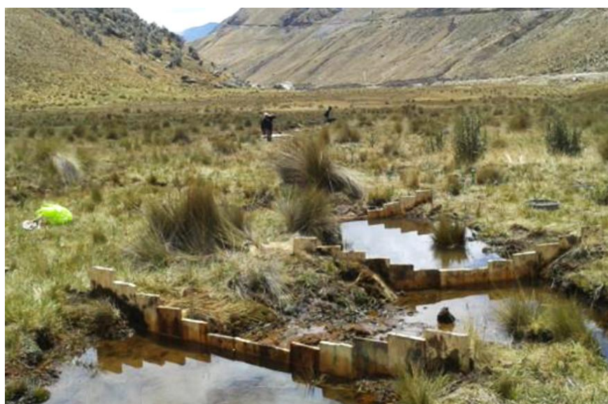
Figure 2. Installation of dams to restore a peat bog (bofedal) in the Pucavado ravine, Huascarán National Park. (© Beatriz Fuentealba)
