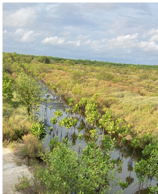
Newly excavated straight and contoured channels to restore hydrology and condition the soil. Active shrimp farms are on the other side of the sanctuary (© WNPS).
