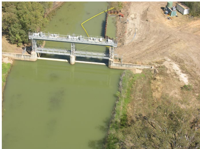
Murray Darling Basin, with water management infrastructure on a river ©Max Finlayson
