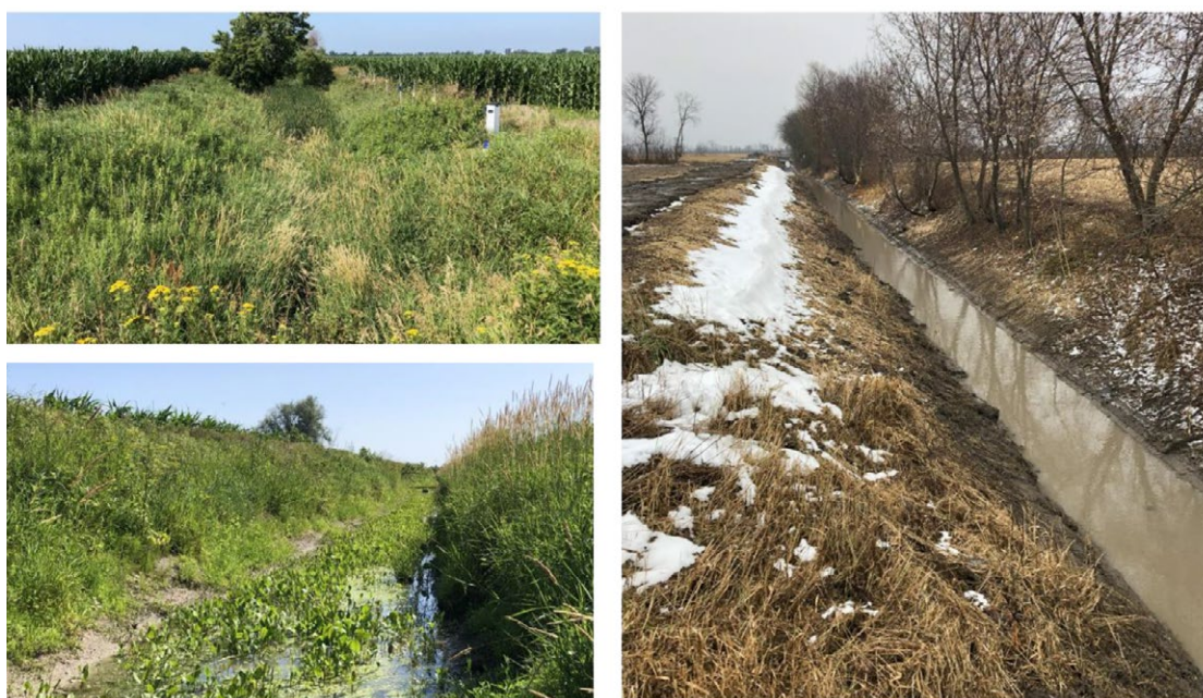
Agricultural drainage ditches, displaying wetland-type features. Clockwise from top left: ditch prior to dredging; ditch after brushing of woody vegetation and dredging; ditch regeneration post-brushing (©Agriculture and Agri-Food Canada)
