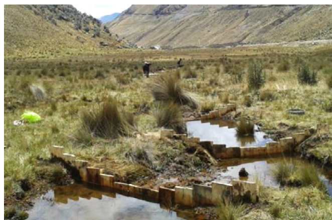
Installation of dams to restore a peat bog (bofedal) in the Pucavado ravine, Huascarán National Park (© Beatriz Fuentealba)
