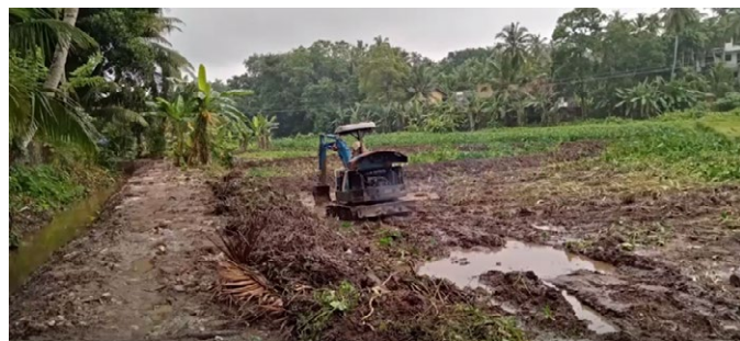
Cleaning and excavation of degraded paddy fields and canals (©Padmini Perera/Manosha Welikala).
